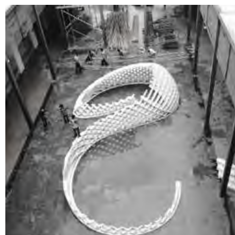
Skeleton of the pavilion ready for cladding
