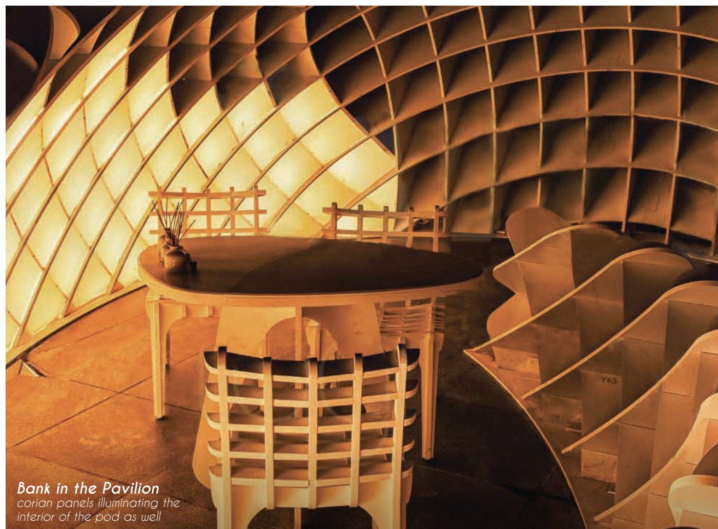
Tactile textured Panels corian allows to pass the light imparting a golden glow to the pod
